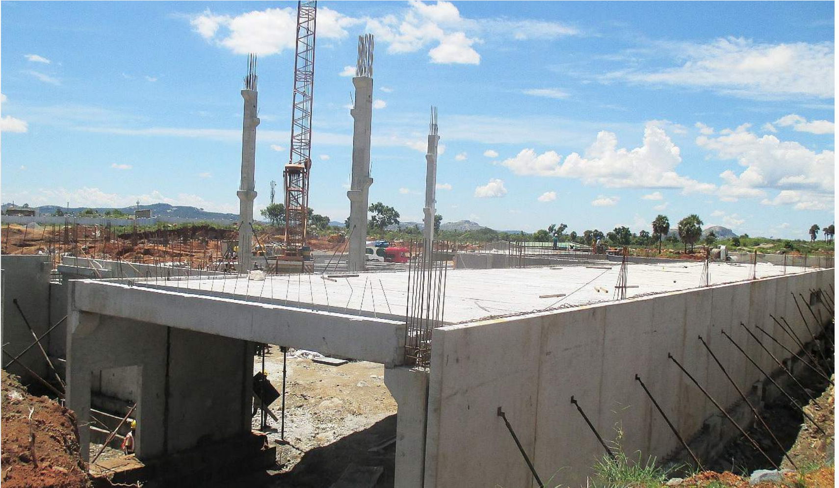
Further Progress at the Stilt floor with the erection of Hollow Core Slabs
