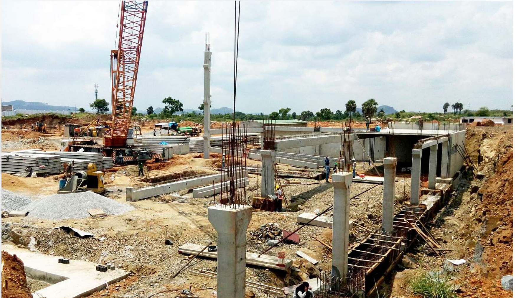
Progress of erection of Prestressed Precast elements - Columns, Beams and Retaining Walls for the Stilt Floor
