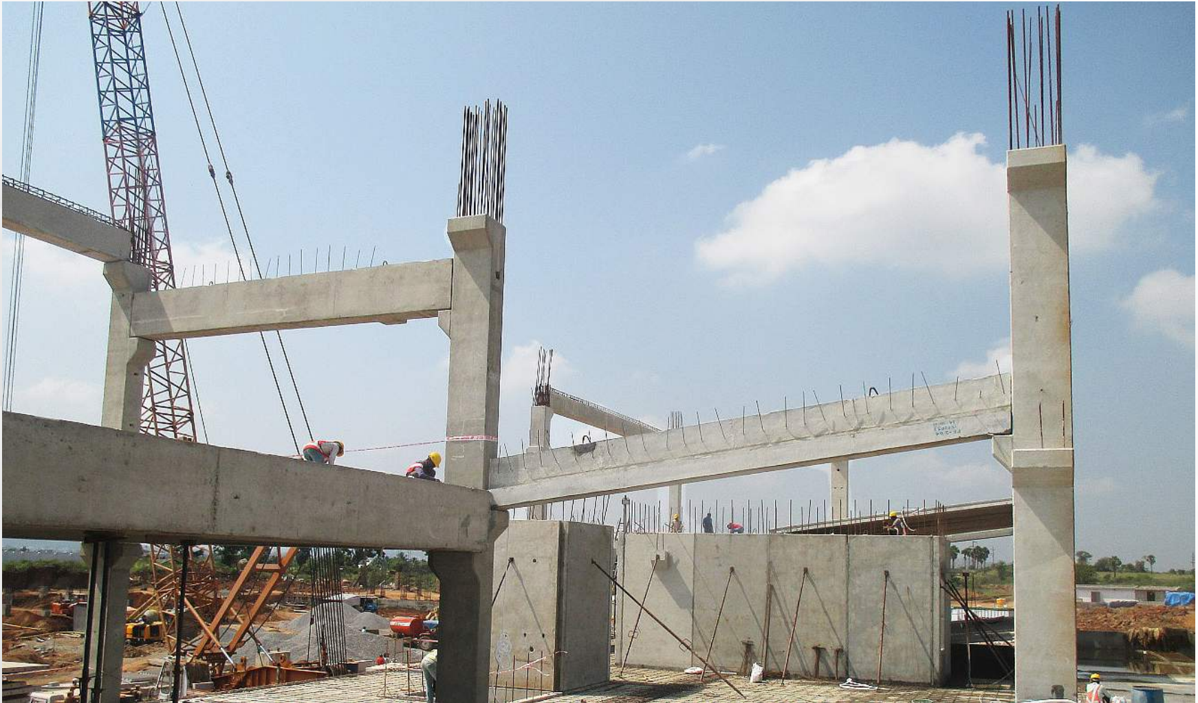
Beams erected at an incline which will later support the flooring of the Lecture Halls on the Ground Floor
