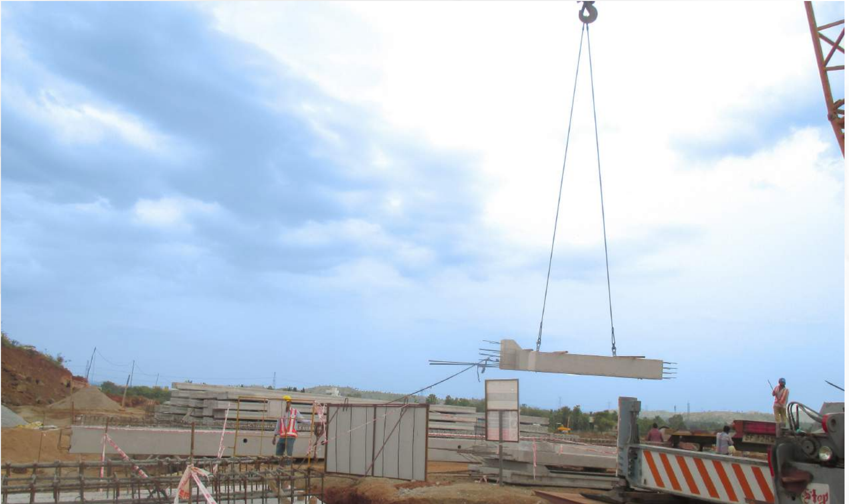
Stacking of the Prestressed Precast Elements on the site as foundation works reach completion
